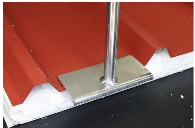
Photo 5 - Place Turn-up Tool centrally over pan
