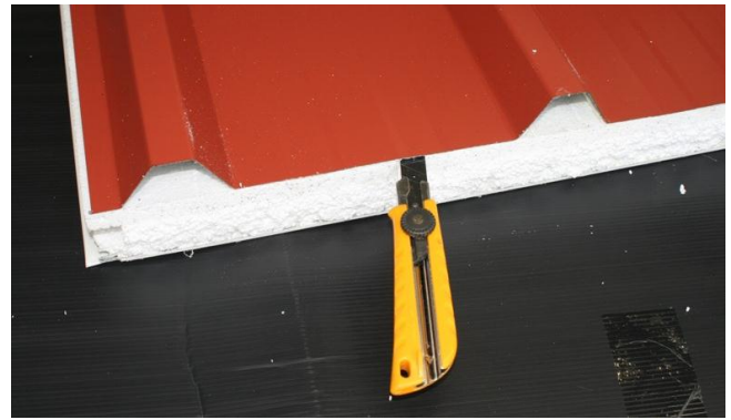
Photo 3 – Cut an EPS wedge from under pan
