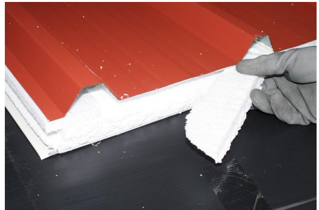
Photo 4 – Remove EPS wedge
