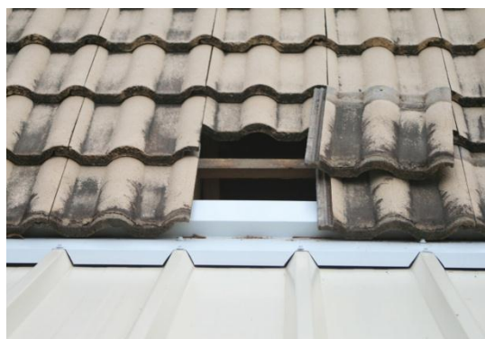
Photo 2 – House roof to Patio flashing
