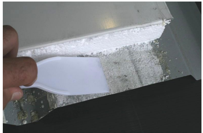
Photo 9 - Remove EPS at gutter end
